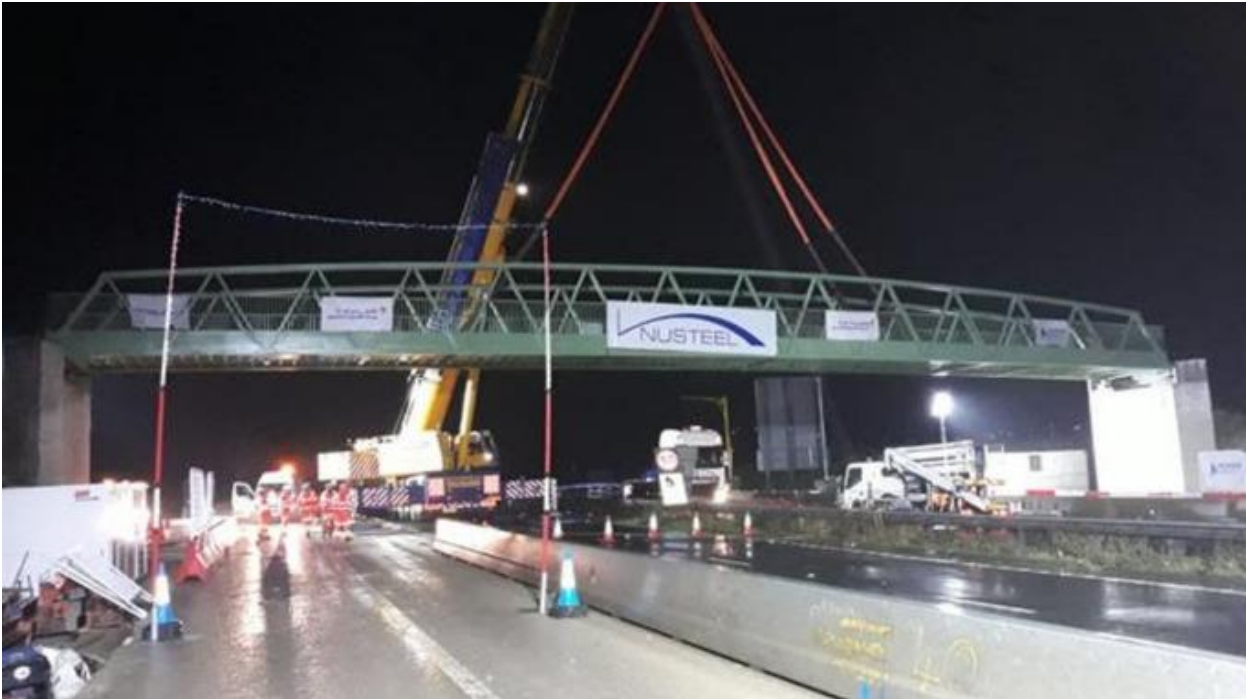
Kingsford Street Footbridge - Central Span Installation.
